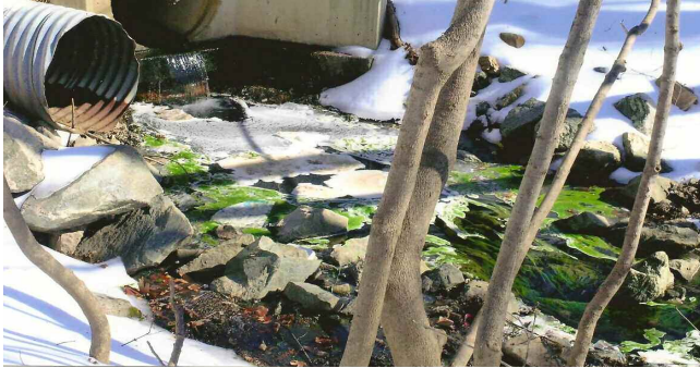
Photo taken on a Crum Creek tributary in winter showing detergent discharge from stormwater outfall and algae in the stream.
